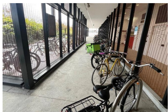
Sydenham Bike Shed (from inside)
