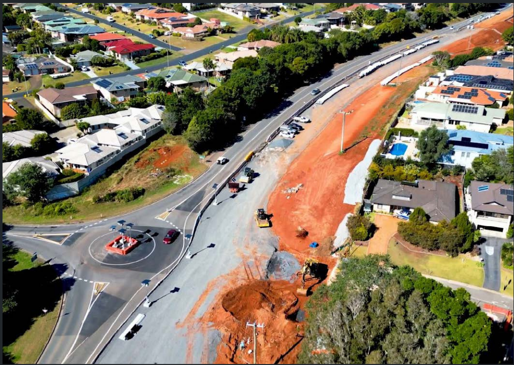
Figure 9. Ocean Drive Infrastructure Project.
